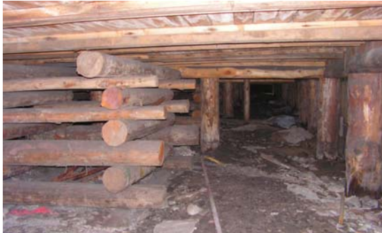
Picture 5.7 Combined Foundation of residential building
