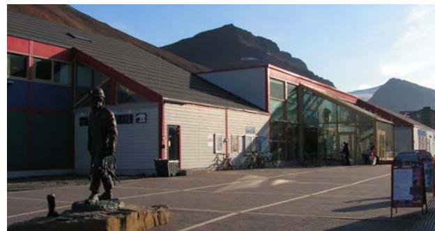
Picture 5.6 Shopping centre with slab foundation
