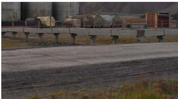
Picture 7.1 Pipeline on concrete piles in Pyramiden
