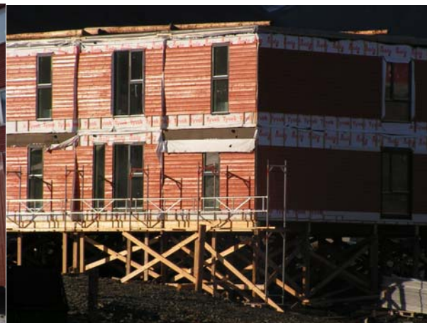
Picture 5.4 Construction site with wooden pile foundations in Longyearbyen
