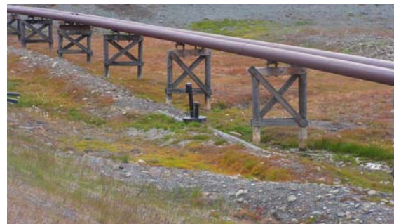
Picture 7.2 Underground pipeline next to a pipeline on wooden piles in Longyearbyen
