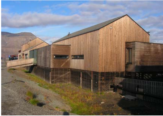
Picture 5.1 Building on wooden piles in Longyearbyen
