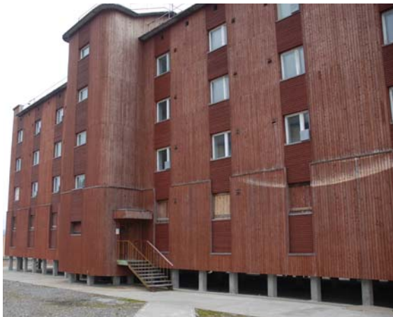
Picture 5.3 Hotel in Pyramiden on concrete piles
