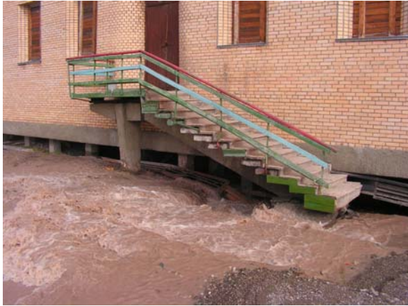
Picture 8.3 (left) River running into the foundation and leading to structural damage of the Madhouse in Pyramiden 2006
