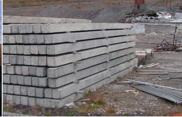
Picture 5.2 Concrete Piles used for foundations in Pyramiden
