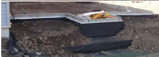
Picture 5.10 Slab foundation of the new cultural house in Longyearbyen during the construction. Cooled concrete slab below the thick insulation and building foundation.
