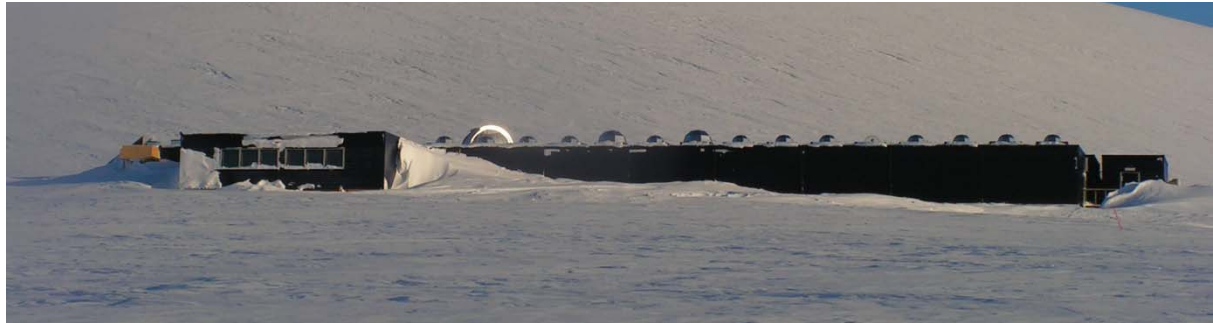
Fig 7: Enormous snow deposition around the Northern Lights station (KHO) near Longyearbyen (The building is built on piles with a length up to 2m)
